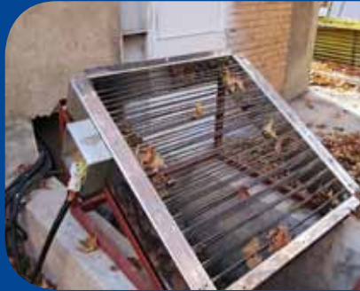
Resistors Bank of Thermal Governor
